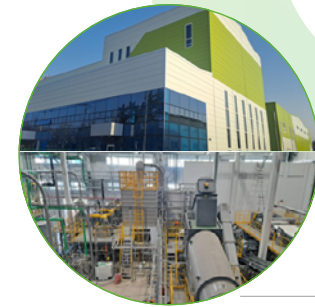
Samyang EcoTech Shihwa Plant
